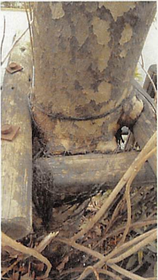
No.27 幹の腐朽
